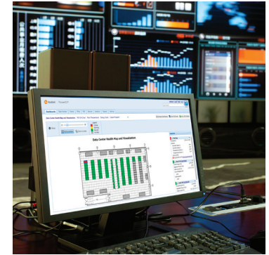
Pillar 5 Safely Manage IT/OT Assets with Remote Monitoring & Switching
