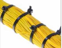
Too many cables bundled together can cause improper bend radius and weight distribution.
