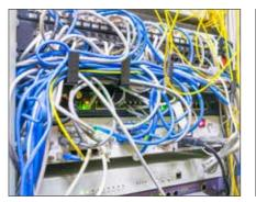
Cables that are mixed and intertwined can cause signal interference.
