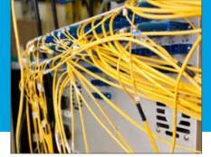
Extensive bending and cables that aren't properly secured can cause signal degradation.
